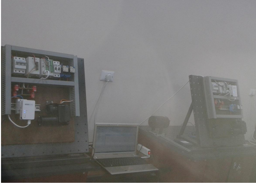
Figure (5. 5):Lab of programmable logic control was connecting using TP-Link Adaptor over PLCC.
